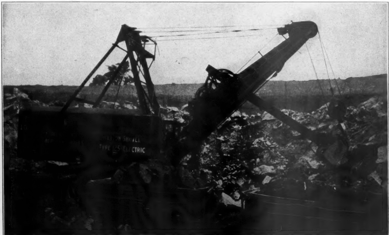
Note the Hoisting Arrangement on the Shovel
